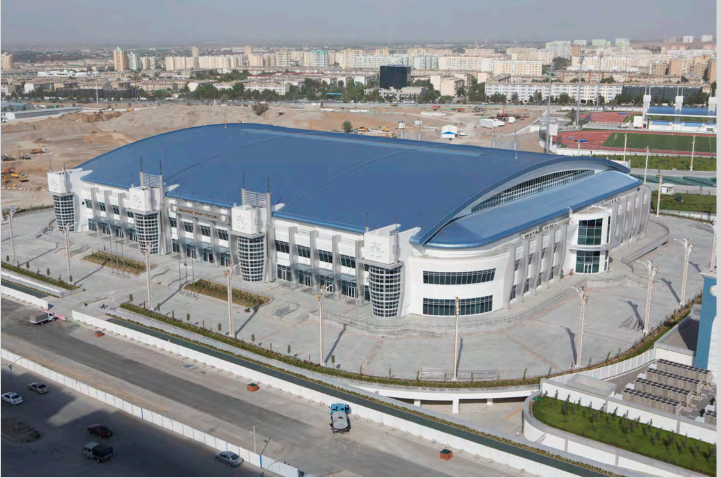
TURKMENISTAN VELEDROM BUILDING
