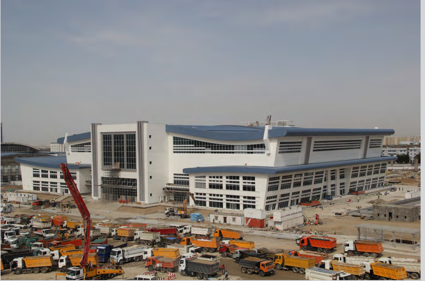
TURKMENISTAN COVERED POOL
