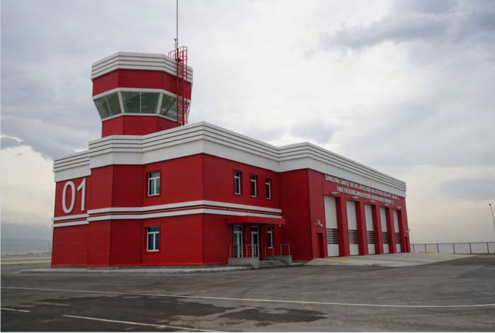
RFF FIRE DEPARTMENT
